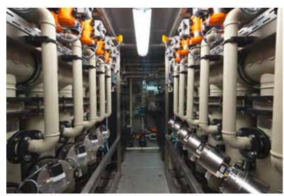
Redundantly equipped ultrafiltration in the OilPaq container
