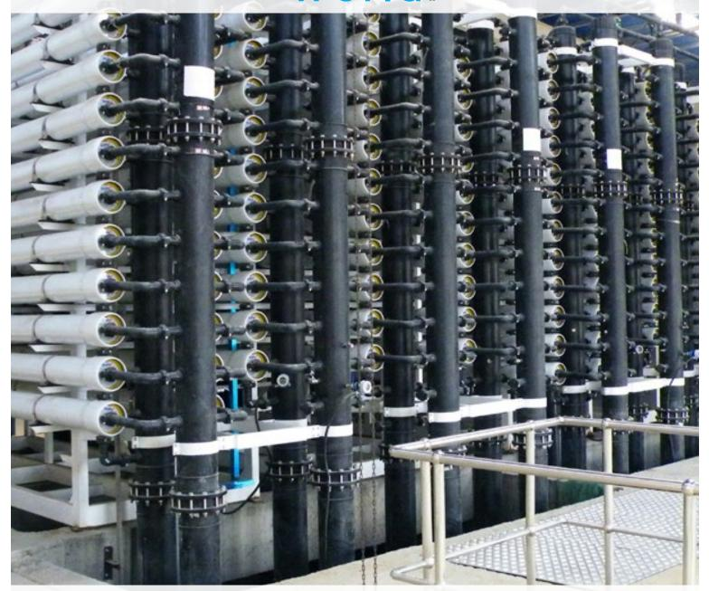
Ultrafiltration Occupies an Established Position In Water Treatment
