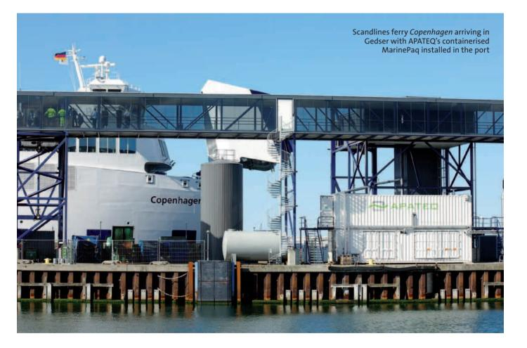
n preparation for the 0.5% sulphur cap agreed by the IMO (International Maritime Organization) for introduction through Marpol Annex VI in 2020, APATEQ has designed and manufactured a new system to treat wastewater from scrubber operation.
