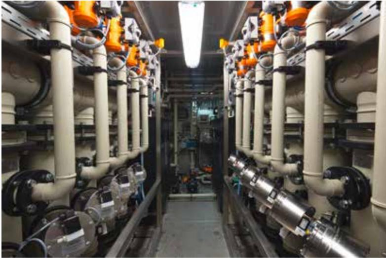
Redundantly equipped ultrafiltration in the OilPaq container
